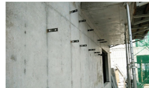
Aluminium Formwork Forming Effect
