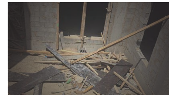
Timber Formwork on Site
