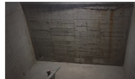
Timber Formwork Forming Effect
