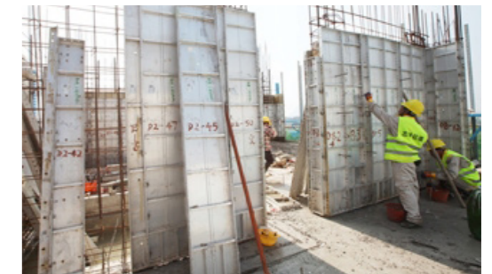
Aluminium Formwork on Site
